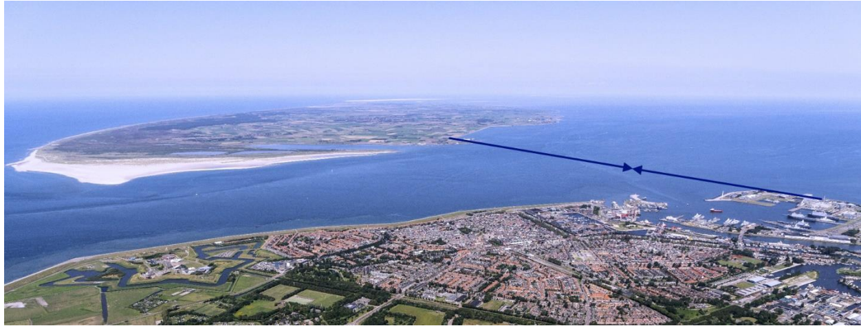
Figure 2. Location of an Intersect Drill with guidance from a Drillguide Gyro Steering Tool
